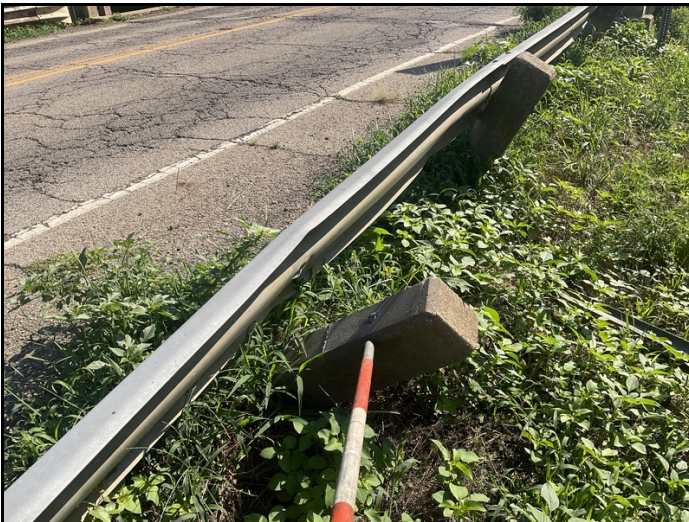
Abutment # 1, right approach railing has collision damage that has fractured two of the railing post and has broken the bolted connection to one of the posts. The railing is leaning away from the roadway.
