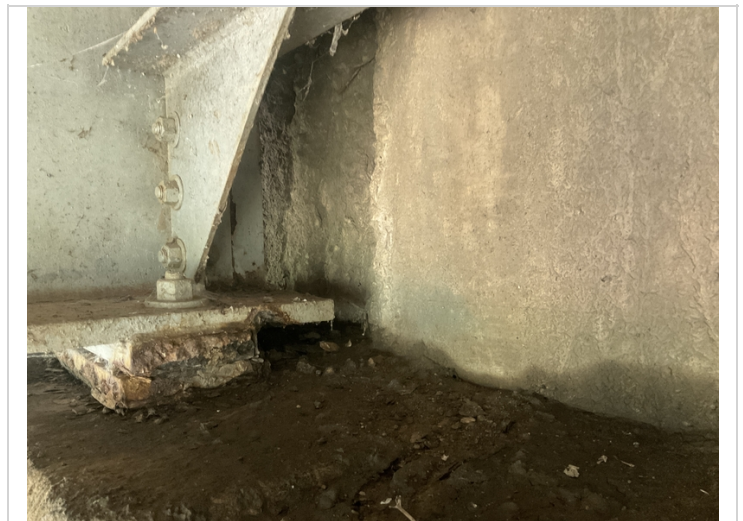
Abutment 2 backwall chipped out to provide additional expansion room
