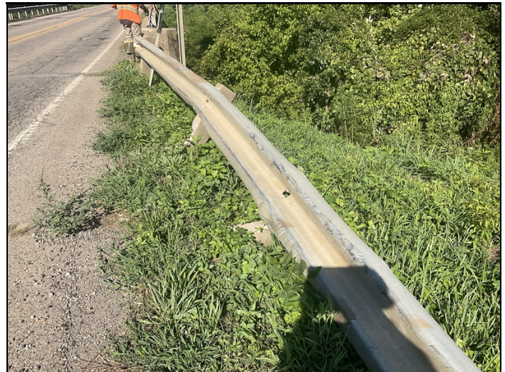
Abutment # 2, left approach railing has collision damage that has fractured two of the railing post.
