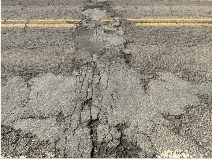
Asphalt breaking apart over bent 3
