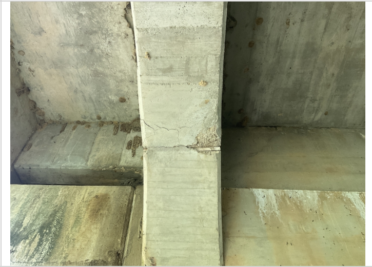
Span # 2, girder/# 4 at bent.# 2 has a delaminated area in the haunch portion of the girder.
