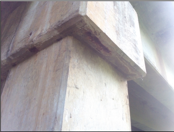
The concrete caps have random areas of shallow spalling with exposed reinforcing steel.
