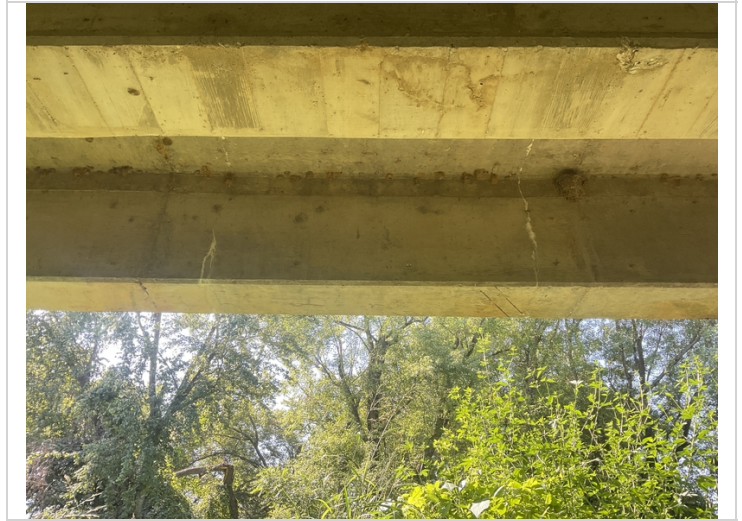
Span 2, girder 5-Vertical cracking with efflorescence
