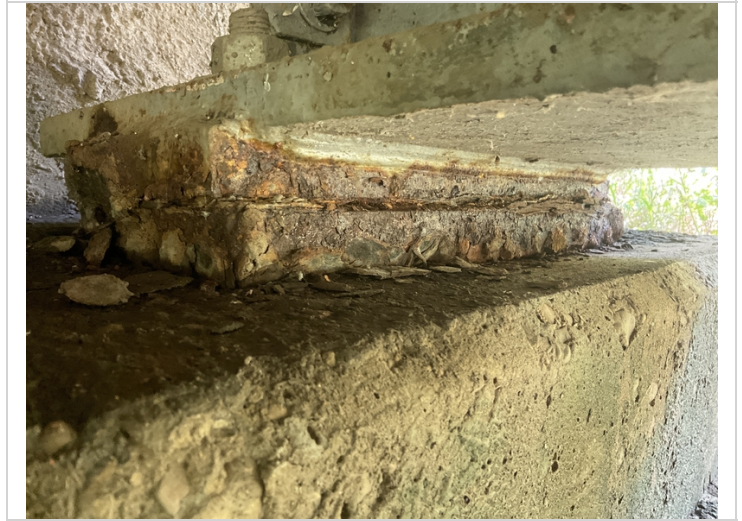
Abutment 2, bearing 4-Corrosion
