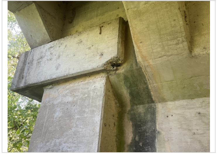
Bent 3 cap backface, left side-Spall with exposed reinforcing steel
