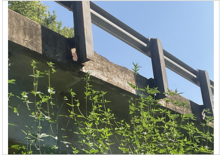
Span 2, right side-Mapcracking with efflorescence
