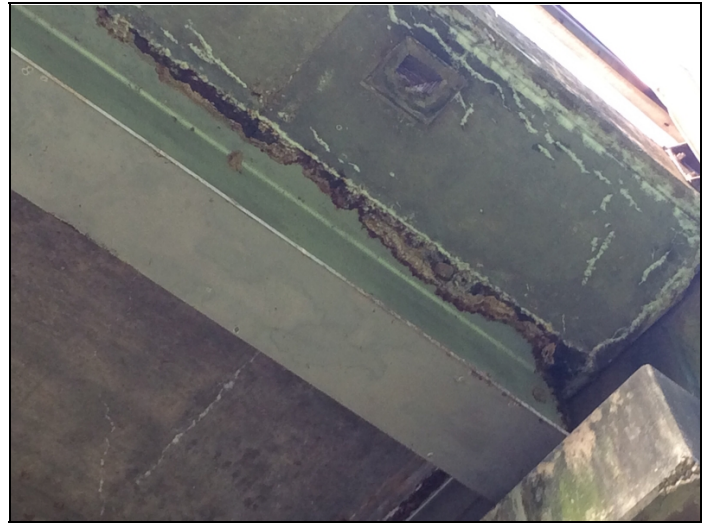
Active corrosion, layers of rust and initial section loss along the top flanges in Span # 3 adjacent to Bent # 3.
