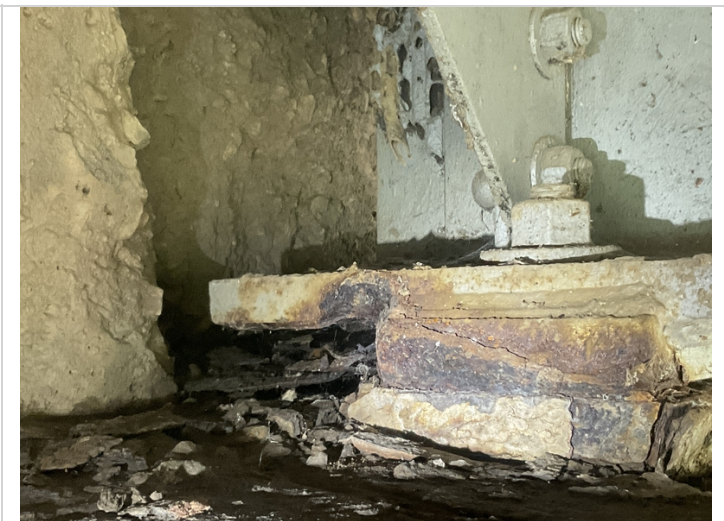
Span # 3, beams # 2 and # 3 have approximately 1/4" section loss to the bottom flange behind the bearing device.
