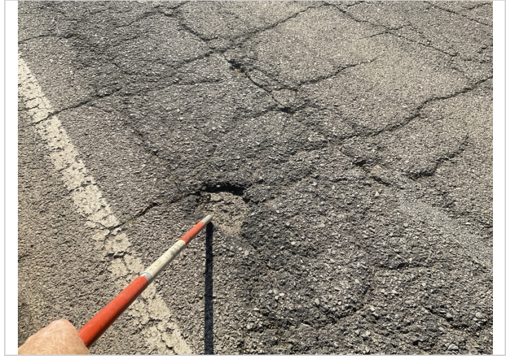
Span 3, left lane-Potholes forming in asphalt wearing surface.
