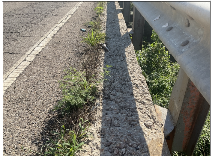
Span # 2, right side-Concrete deterioration to curb.
