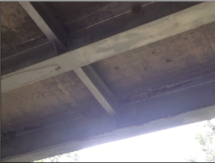
The steel beams have areas of corrosion with flaking rust. Beam # 4 is the most notable area with numerous areas of corrosion with flaking rust along the interior and exterior sides of the beam.
