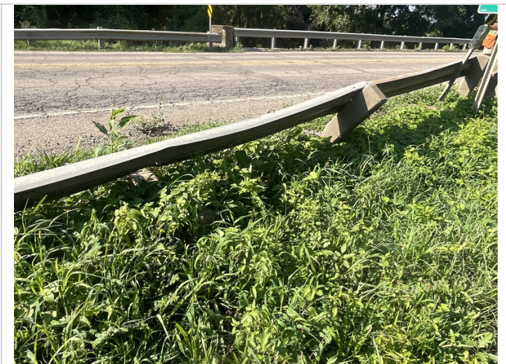
Abutment # 2, left approach railing has collision damage that has fractured two of the railing post.
