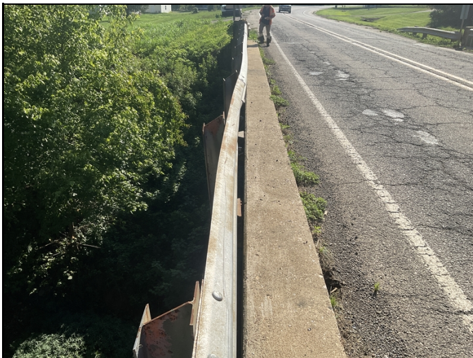
Span 3, left railing-Collision damage.
