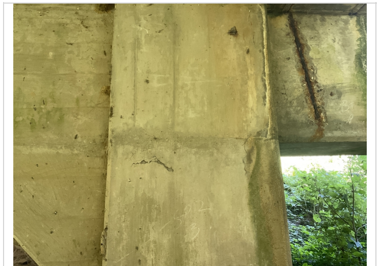
Bent # 2, column # 2 aheadface has vertical cracking and minor delaminated area at cap juncture.
