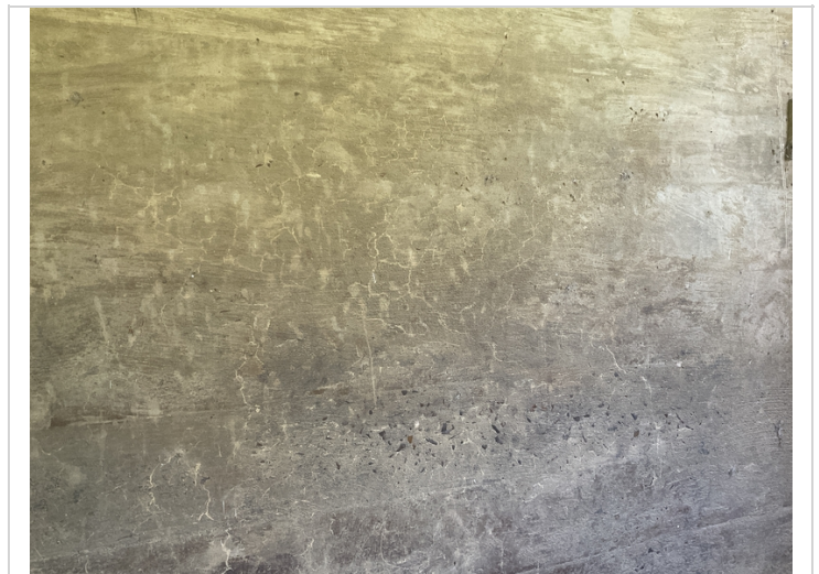
Bent 3 web wall-Superficial mapcracking
