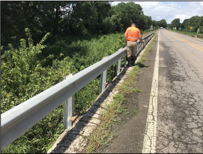
Right curb-Concrete deterioration with exposed reinforcing steel.
