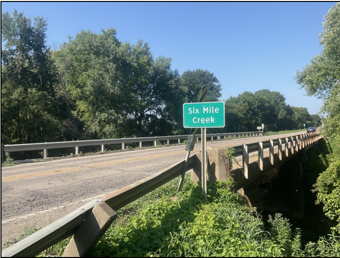
The flare board sign on the left side of abutment # 2 is twisted away from the roadway.
