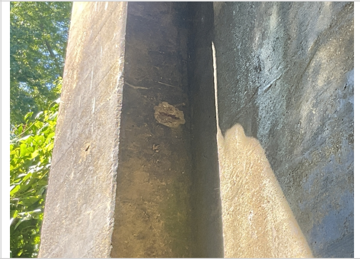
Bent 3, column 1 aheadface-5" spall with exposed reinforcing steel
