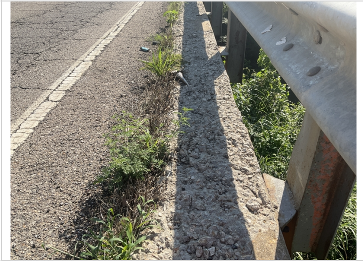
Span 2, right side-Concrete deterioration to curb
