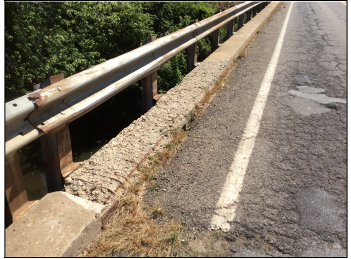
Left concrete curb-Deterioration with exposed reinforcing steel.
