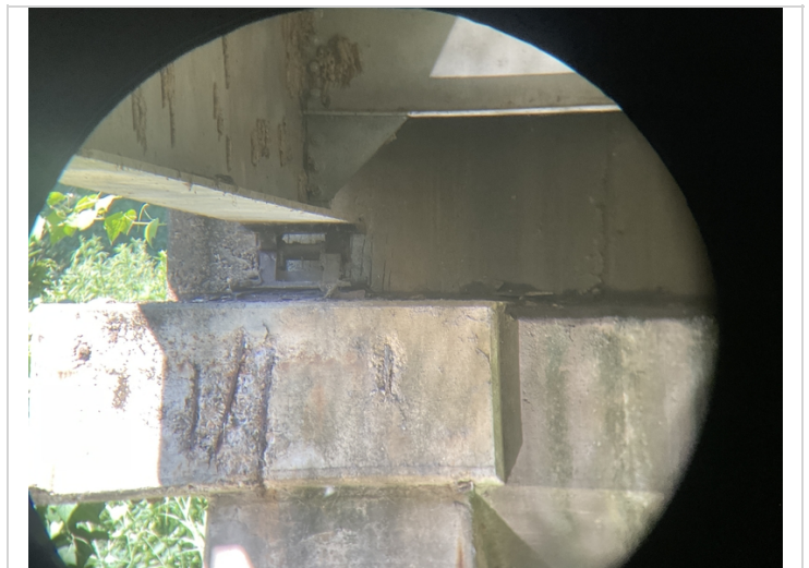
Movable bearings at bent 3-Corrosion with pack rust between rockers and masonry plates.
