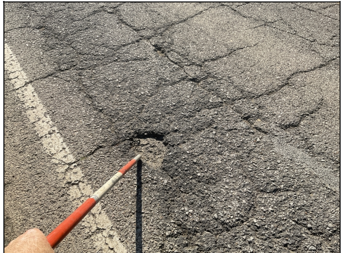
Span # 3, left lane-Potholes forming in asphalt wearing surface.
