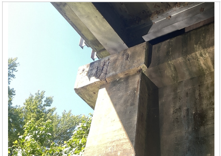
Bent 3 cap aheadface, right side-Spalling with exposed reinforcing steel
