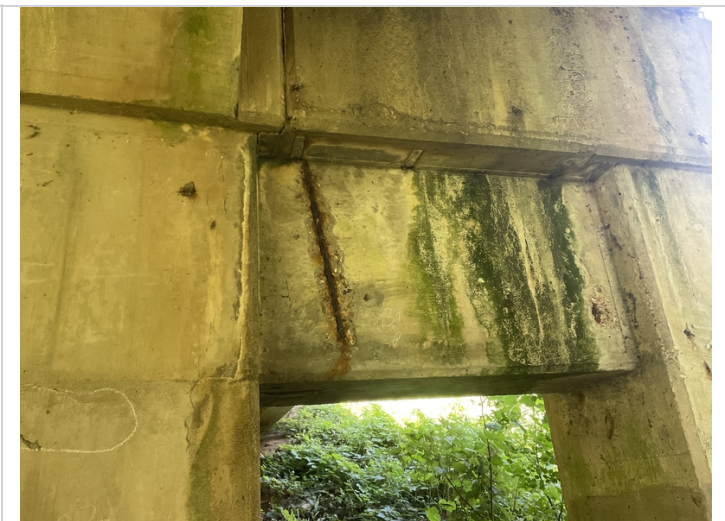
Bent 2 cap haunch, left side-Spalling with exposed reinforcing steel in ahead side
