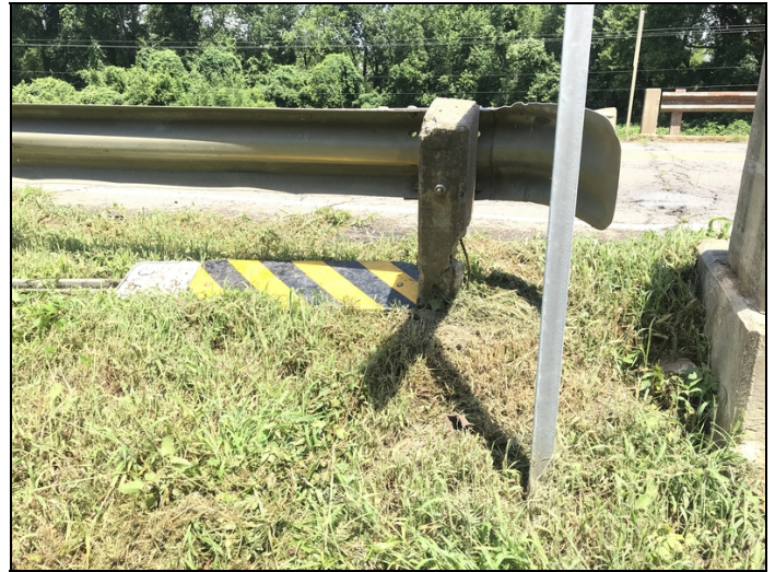
Fractured approach guardrail post.
