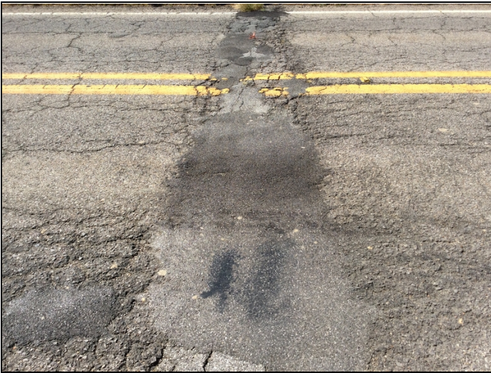
Bent # 3 asphalt breaking apart over the bent.
