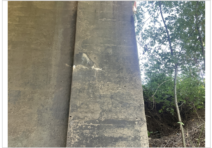
Bent 3, columns # 1 and 2 have a hairline horizontal crack with light efflorescence in the aheadface mid-way up the column.
