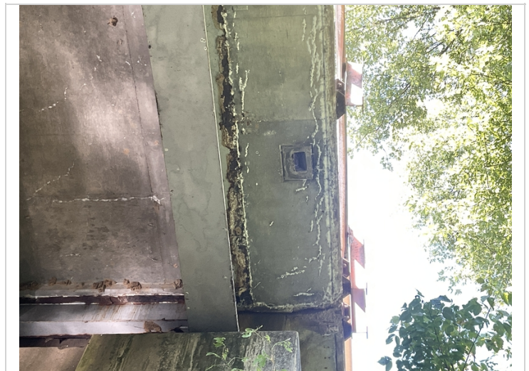
Span 3, right side-Mapcracking with efflorescence in deck overhang
