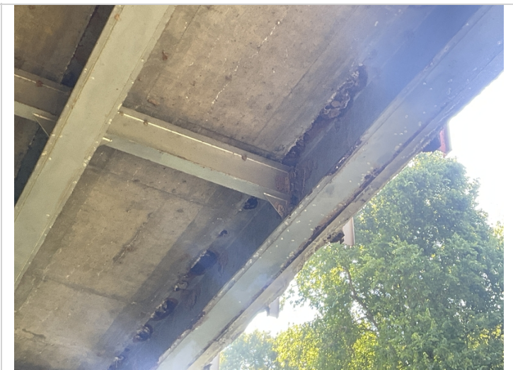
Span 3, beam # 4 has numerous areas of corrosion to the interior and exterior sides of the top and bottom flanges.
