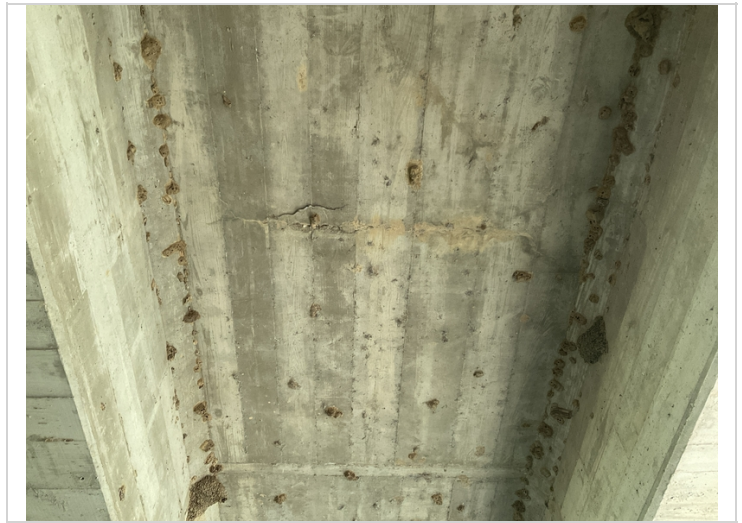
Span 2, bay 3-Transverse crack in deck undersurface with shallow spalling
