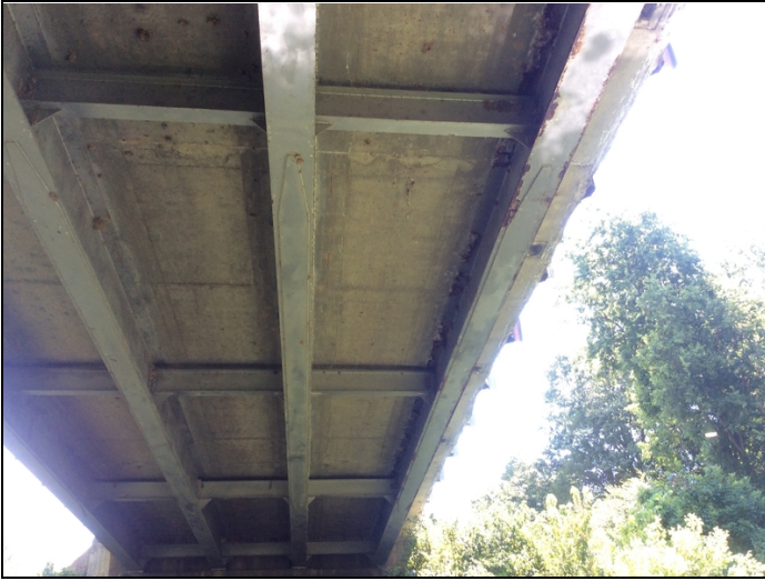
Span # 3 efflorescence leaching through the deck.
