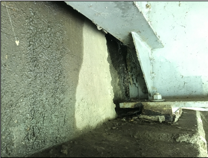
Active corrosion in beam ends and bearings at abutment # 2.
