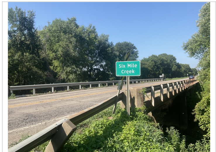
The flare board sign on the left side of abutment # 2 is twisted away from the roadway.
