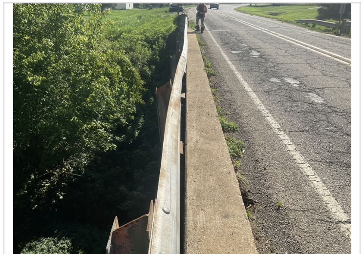
Span 3, right railing-Collision damage
