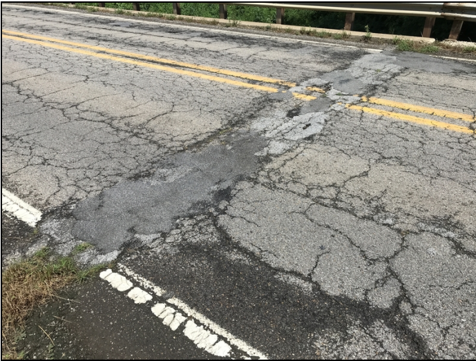
Asphalt wearing surface over bent # 3 is breaking apart.
