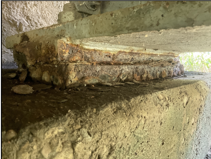
Abutment # 2, bearing # 4-Corrosion.
