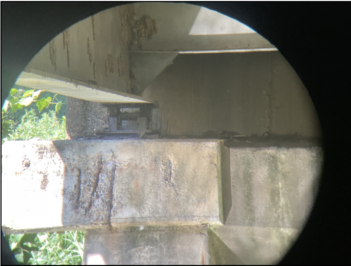
Movable bearings at bent # 3-Corrosion with pack rust between rockers and masonry plates.
