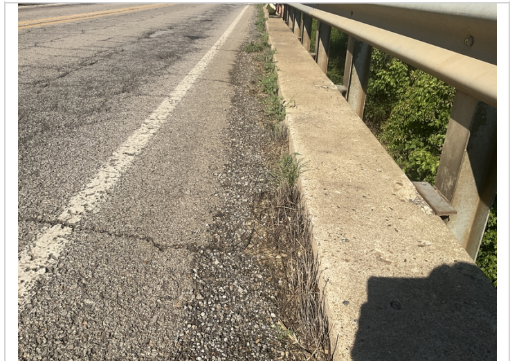
Dirt and debris in gutters
