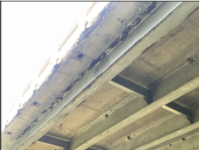
Span 3, beam # 4 has numerous areas of corrosion to the interior and exterior sides of the top and bottom flanges.
