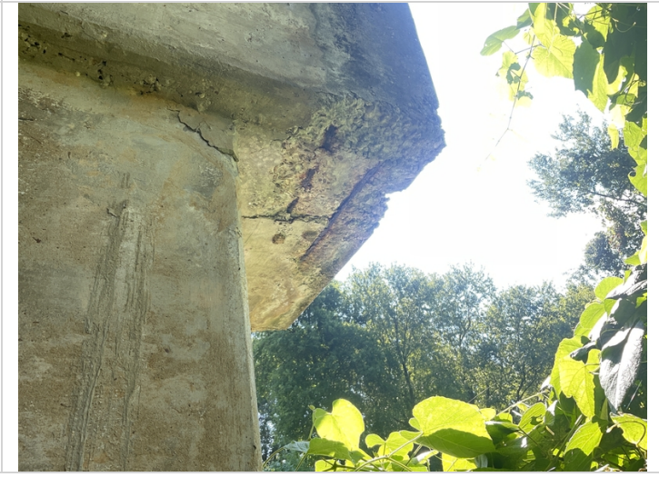
Bent 3 cap, right side-Spalling with exposed reinforcing steel
