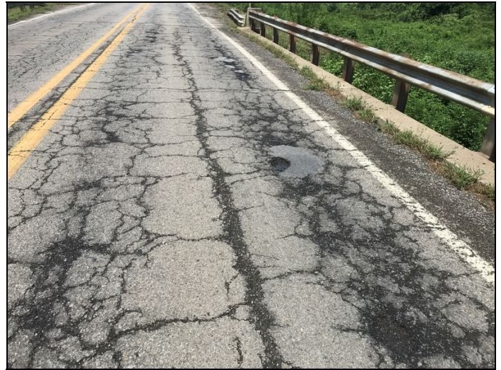
Asphalt wearing surface of the deck is breaking apart in the wheel paths and over the intermediate bents with potholes forming. The asphalt wearing surface has heavy map cracking throughout.
