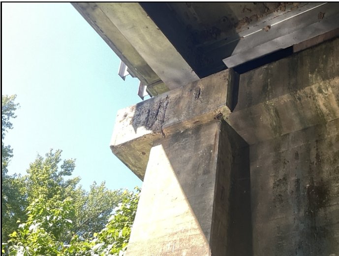
Bent # 3 cap aheadface, right side-Spalling with exposed reinforcing steel.
