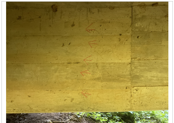
Typical of vertical flexure cracks in girders
