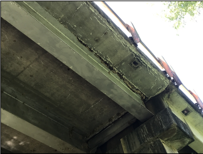
Span # 3, beam # 1 at bent # 3-Active corrosion in the top flange with layers of flaking rust.
