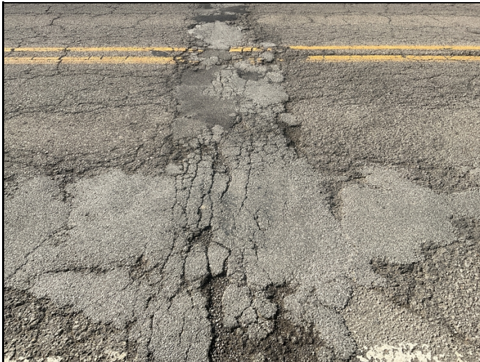
Asphalt breaking apart over bent # 3.
