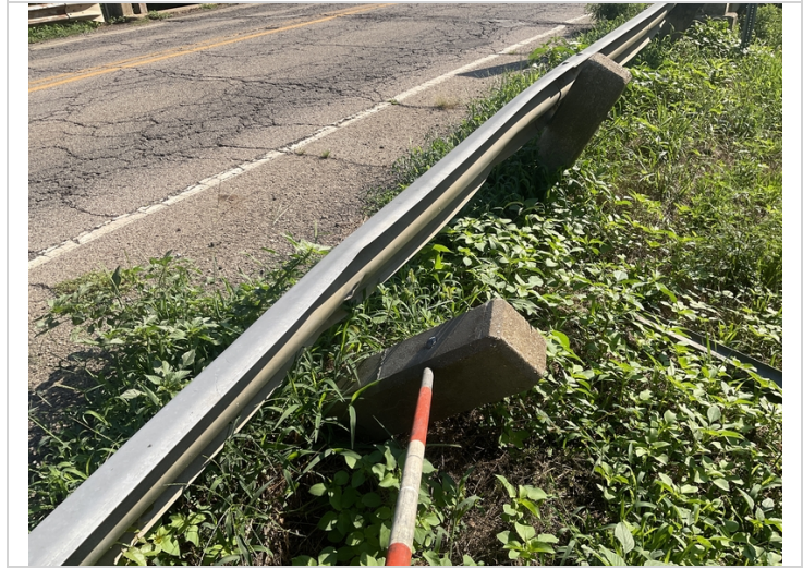
Abutment # 1, right approach railing has collision damage that has broken the bolted connection to one of the posts and caused the railing and posts to lean away from the roadway.
