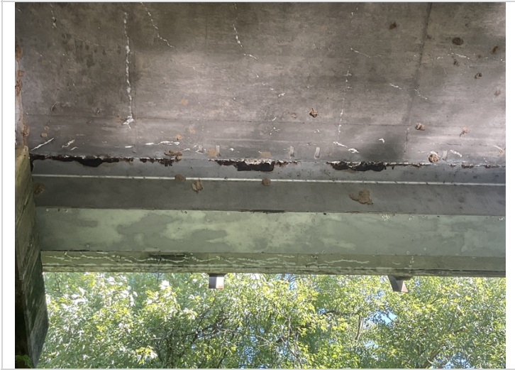
Span 3, beam 1 at bent 3-Corrosion to top flange
