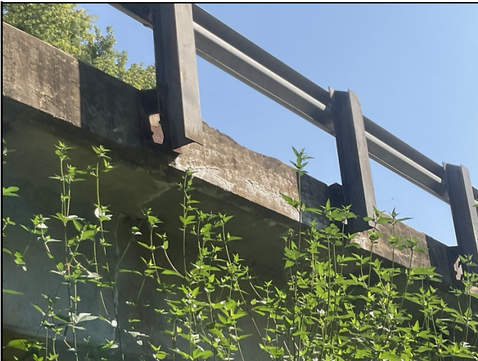
Span # 2, right side-Mapcracking with efflorescence.
